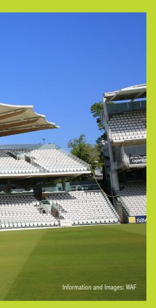
the seating tier, radiating dramatically from the corner of the Ground. The overall form of the main roof is reminiscent of an elegantly spreading palm leaf, delicately folded, so that rainwater runs back to the rear edge of the roof.
